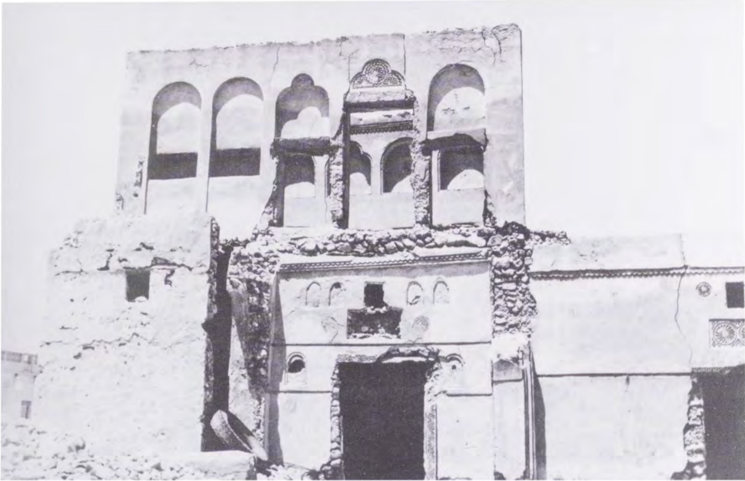
(Fig. 16) : Sheikh Hamad Bin Abdullah's residence before restoration.
